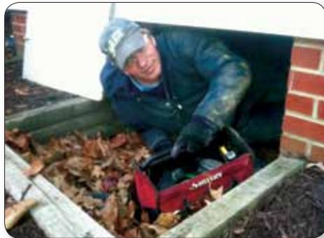
Roger Stigall, residential HVAC service technician, crawls under a house during a service call.
