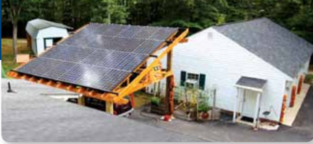
James River Air specializes in energy services including solar solutions. Pictured above is a solar panel array over a car port.
